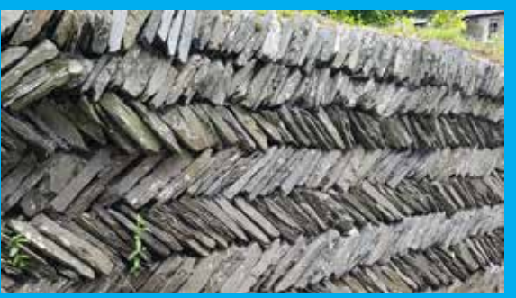
A Cornish hedge is a stone-faced earth bank, often with bushes or trees growing along the top. It is not known as a hedgerow or wall.
